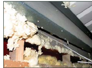
Poor air sealing examples
