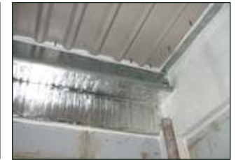
Remedial air sealing examples
