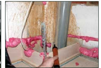
Poor air sealing examples
