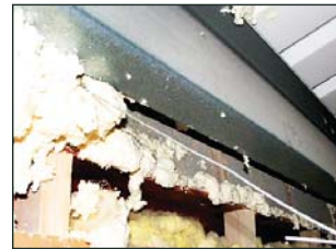
Poor air sealing examples
